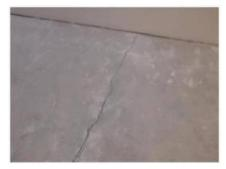
The concrete floor shows signs of minor cracking. Please refer to section of this report - CRACKING OF BUILDING ELEMENTS for additional details.
